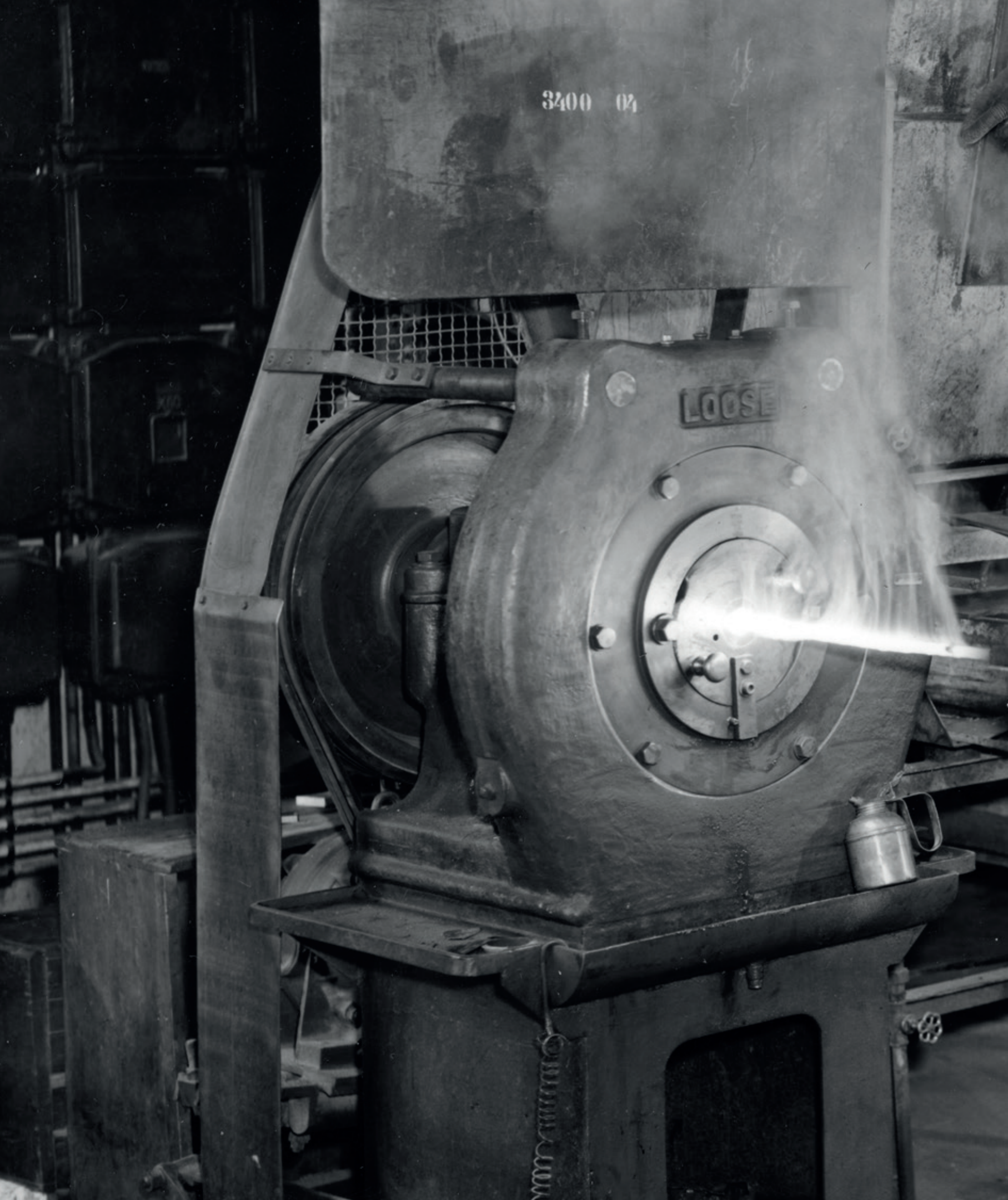
Hands-on work at the machine: this skilled Plansee employee forges molybdenum or tungsten rods at the radial swaging machine. The rods are later used to produce wires, glass melting electrodes, or cathodes for cinema lamps.
