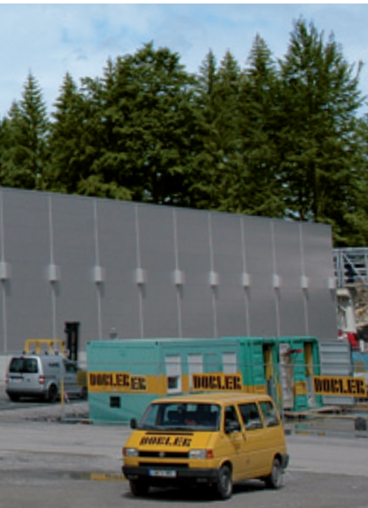
Major investments: The new production plant at the Reutte site in Austria amounts to more than 100,000 square feet.
