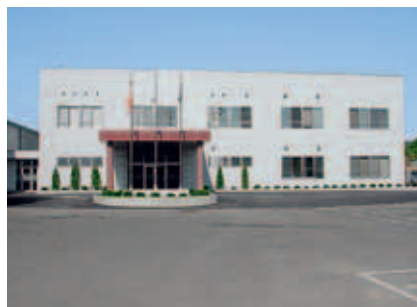
Capacity increased: New production facilities at Vacs Precision in Japan.
