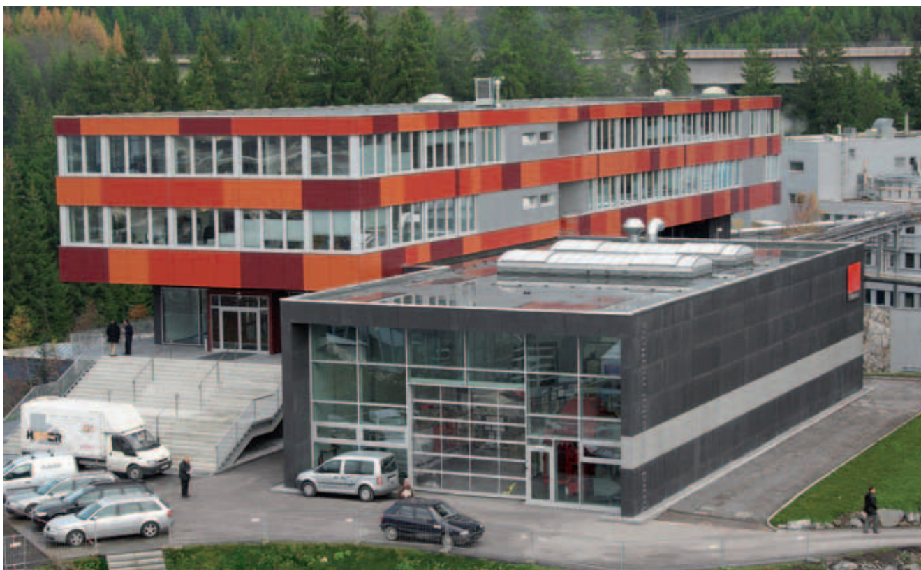
Ceratizit in Reutte, Austria: New office building and Tooling Academy (right).
