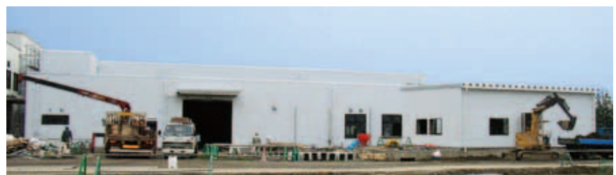
New building at Fujioka plant to increase production facilities.
